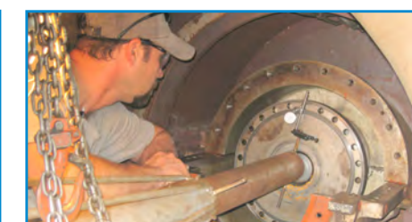
GE Frame 5 Turbine Rotor Alignment
